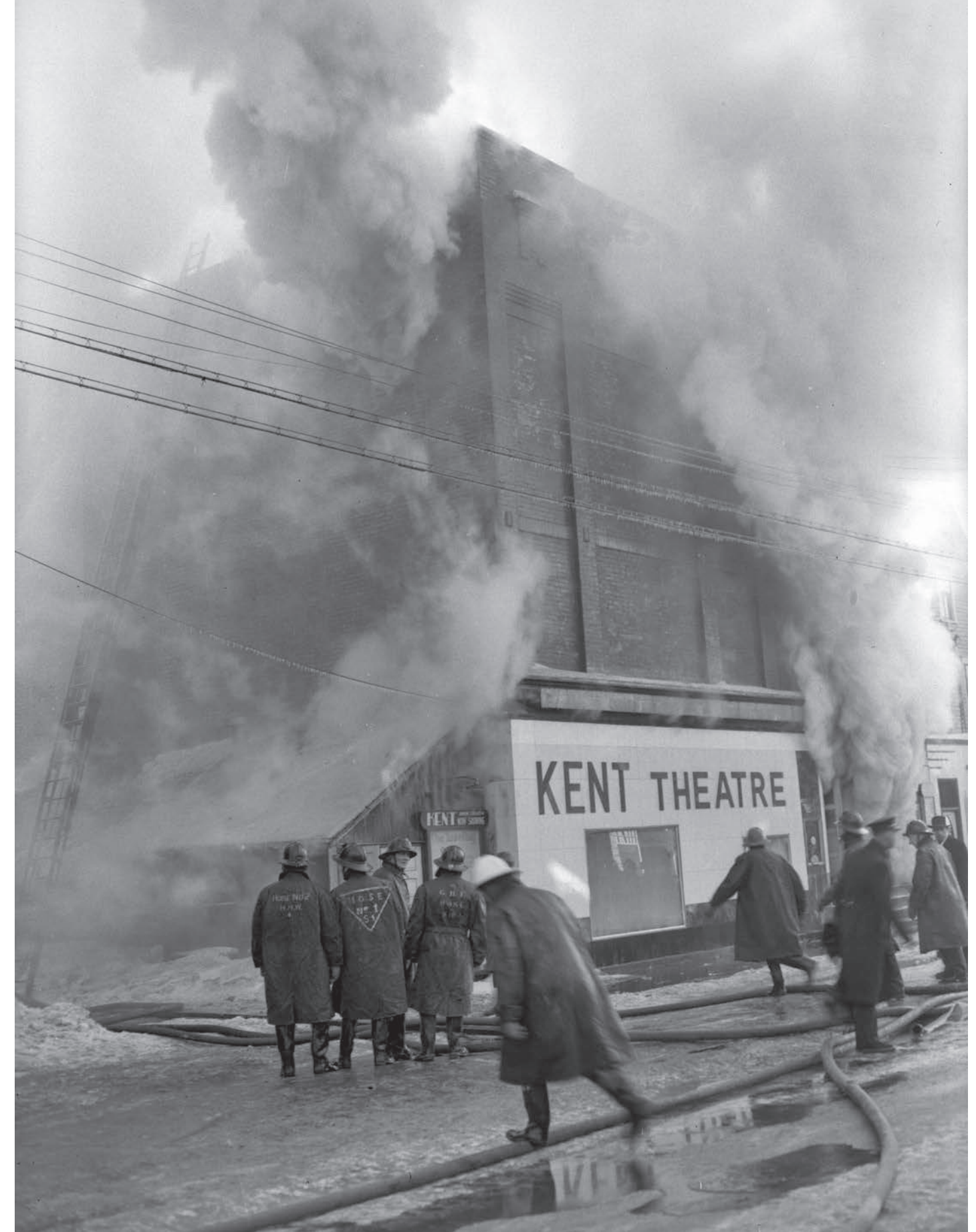
Members of the Moncton Fire Department (firefighters) putting out a fire at the Kent Theatre. The manager LR Conrad safely evacuated 250 kids and 100 adults, no loss of life or injury. February 7 th , 1948. (P913-1)
